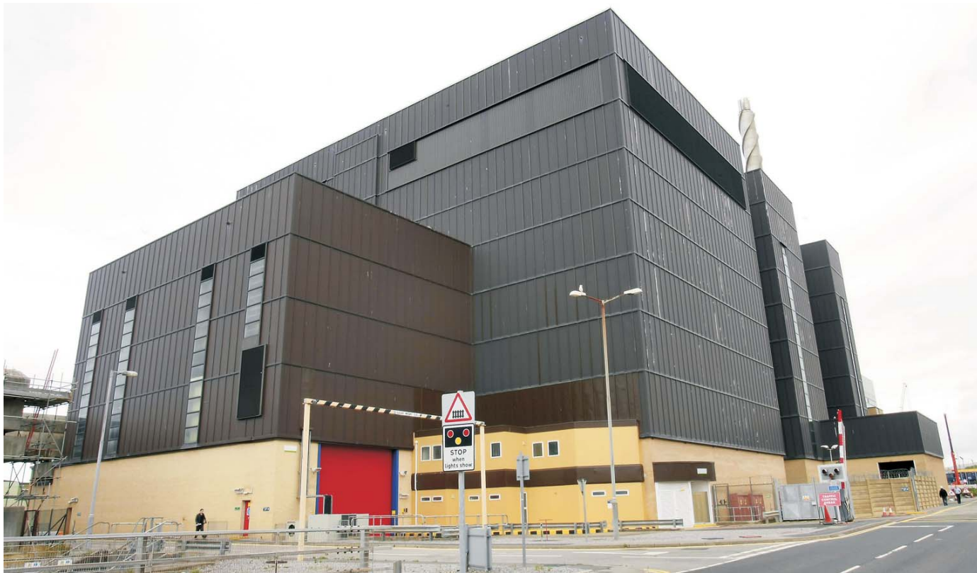
The Residue Export Facility at Sellafield
