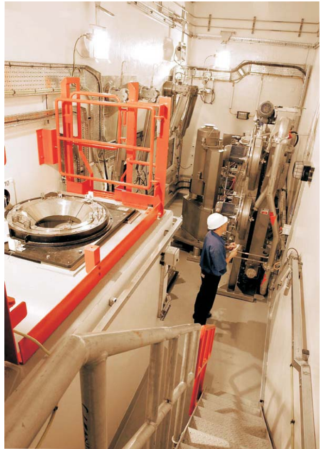
An operator carries out final commissioning inspections in the cleaning cell
