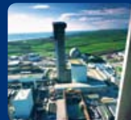
Legacy reactor exhaust stacks
