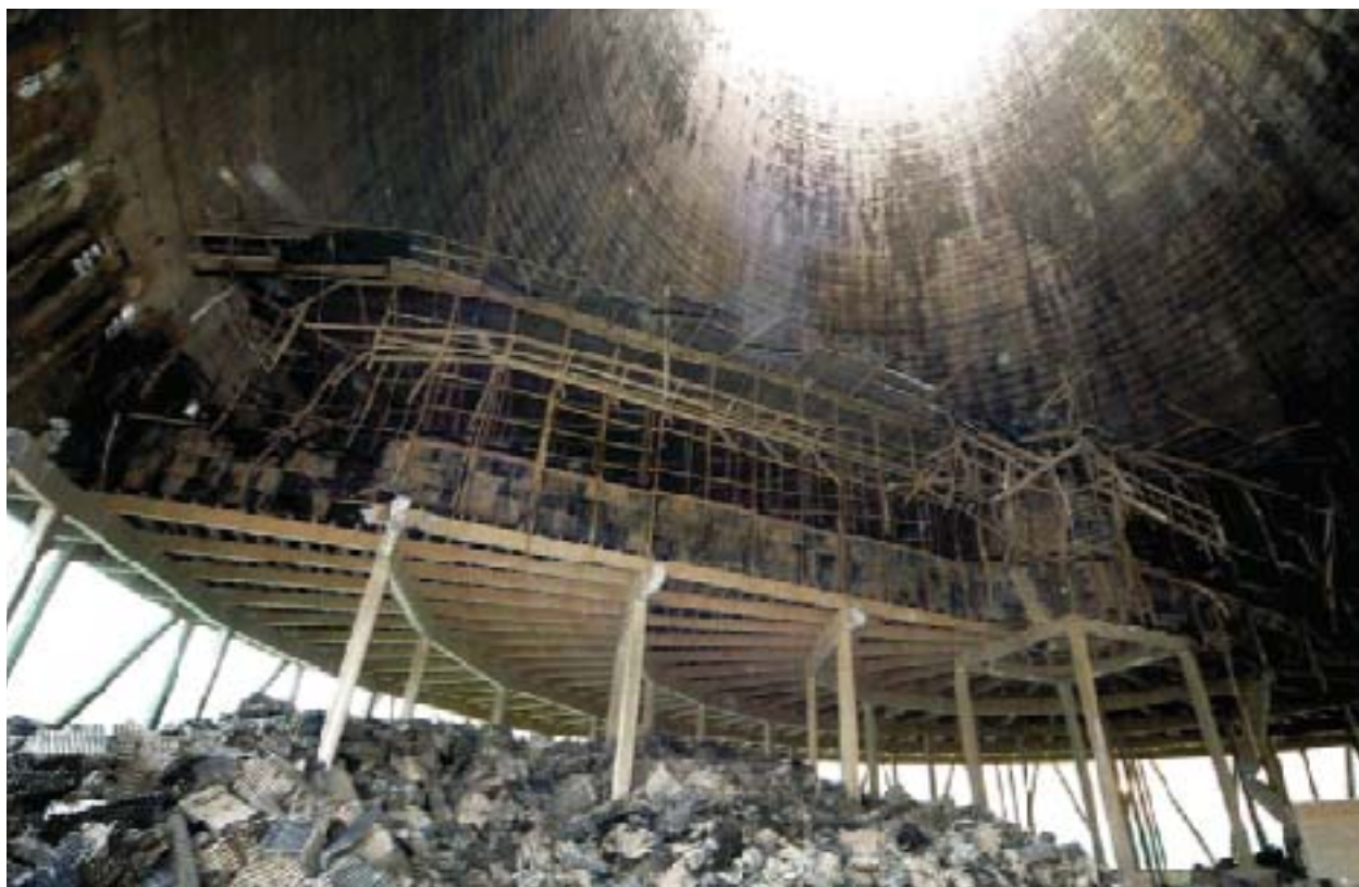
Photograph of tower interior showing various layers of internal structure.
